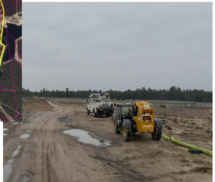
Construction for industrial solar on Priority Habitat, July 2021
